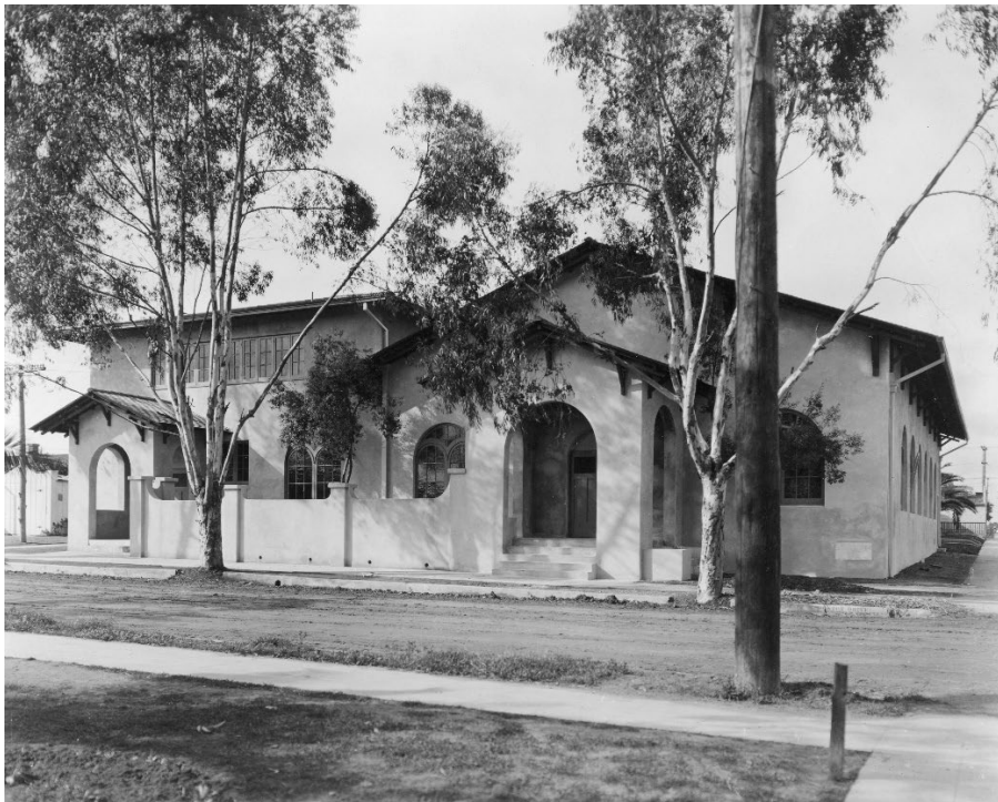
Figure 6 Mission Hills Congregational Church, 4170 Jackdaw Street (Arnold and Choate's Addition), 1928 (San Diego History Center)
